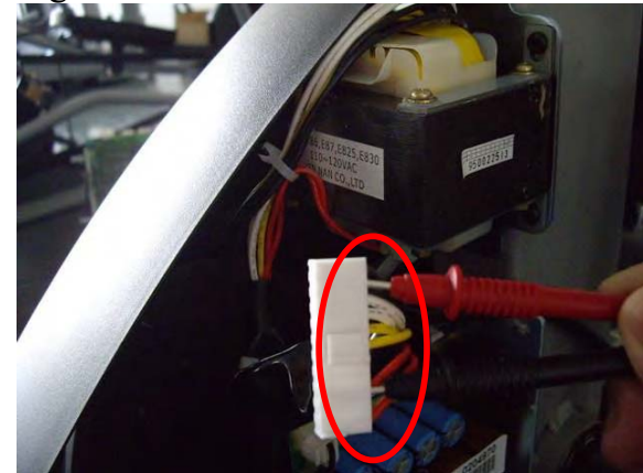
Fig. 2. Electrical Short Test
